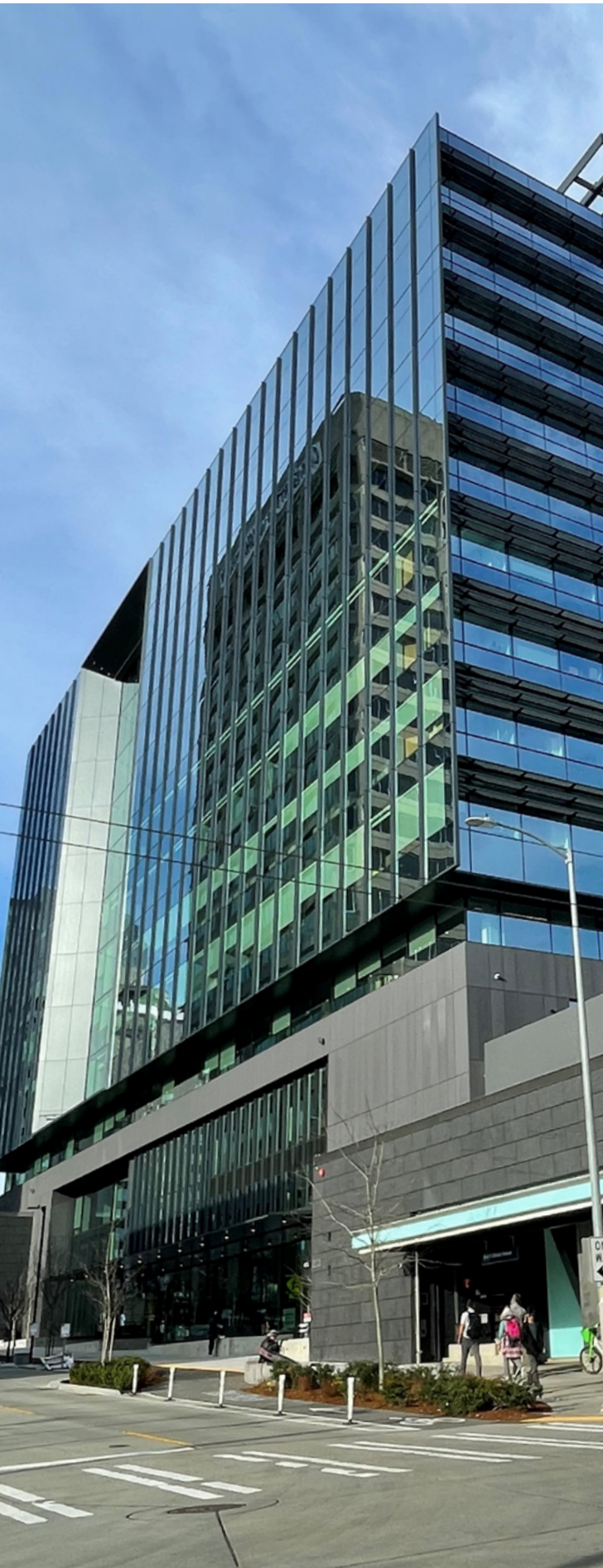
Image: The University of Washington Gateway Building as an example of station overbuild. Image courtesy of Sound Transit.
