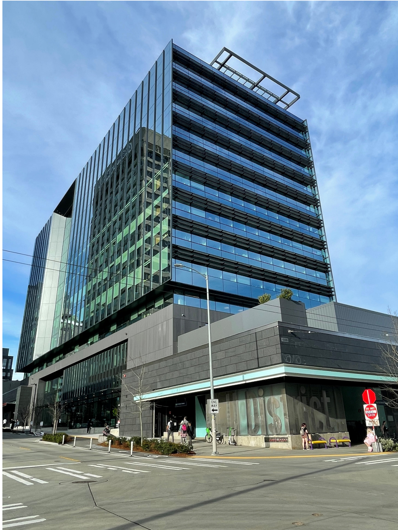
Gateway Building above U District Station, completed 2024. Source: Sound Transit
