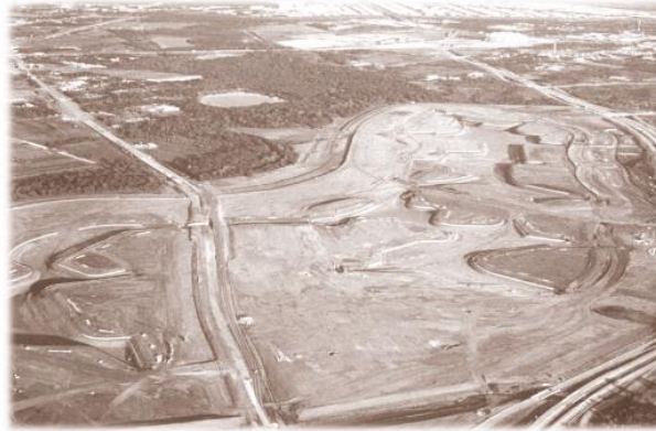
Lake Carolyn during the initial phase of excavation.
