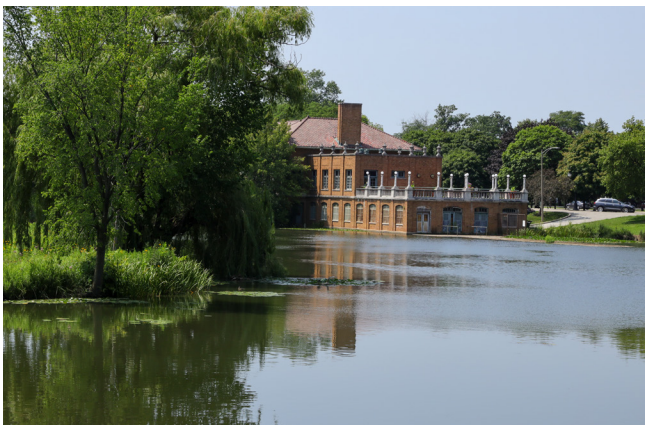
Spanish style refectory and lagoons in Columbus Park located at the southern edge of the study corridor.
