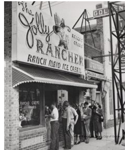
The Jolly Rancher made candy in Wheat Ridge until 2002 and operated this retail store in nearby Golden. Today the cleared 14-acre site is key to the station area's future.
