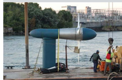
Verdant Power’s Roosevelt Island Tidal Energy (RITE) project in the East Channel of the East River, New York City. Source: TETHYS.pnnl.gov.
