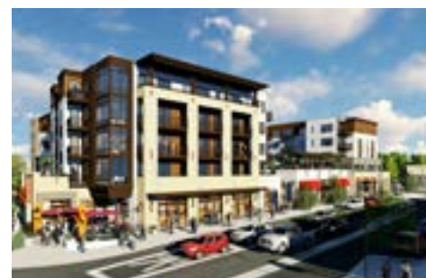
100 Main Under Construction Developed by: Streetlights Residential
