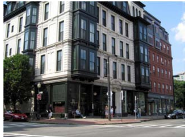
Plan for the long term and appropriate densities. This Boston mixed-use property illustrates model housing densities the City should consider for the future
