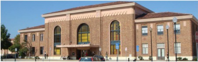
The existing historical Diridon Station
