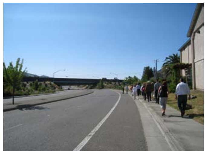
Existing access to station along Citrus Fair Drive
