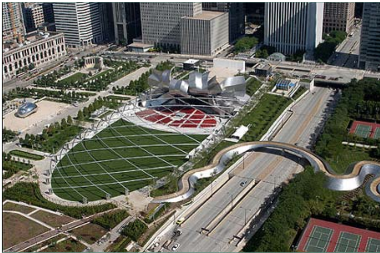
Millennium Park in Chicago presents an example of air rights opportunities realized with a 24.5 acre park was built over commuter railyards. Source: Chicago Convention and Tourism Bureau
