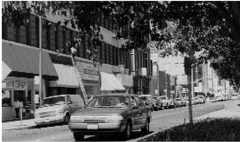
Disinvestment downtown over the last 20 years has left many buildings underused or vacant.
