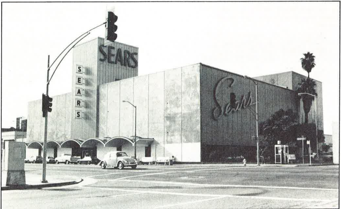
Sears store awaiting remodeling.
