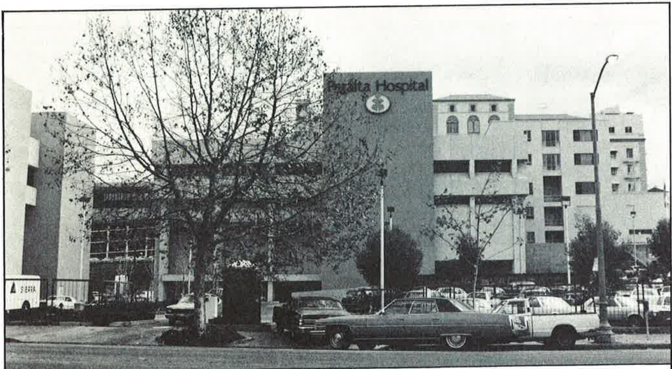
View of Peralta Hospital from Telegraph.
