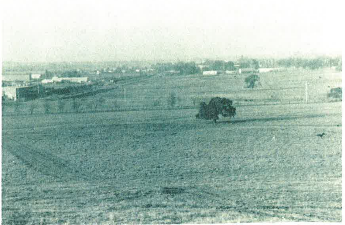
The site looking north with Kaiser plant on the left.
