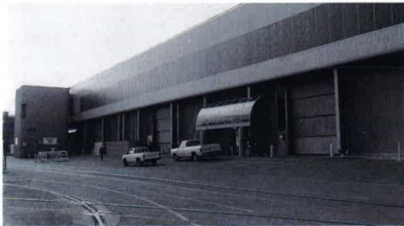
The Pipe and Copper Shop (Building 126) was built in 1985 and contains 130,000 square feet.
