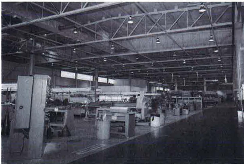
The 105,600-square-foot Sheet Metal Shop (Building 1310) was built in 1972 and is equipped with state-of-the-art machinery.
