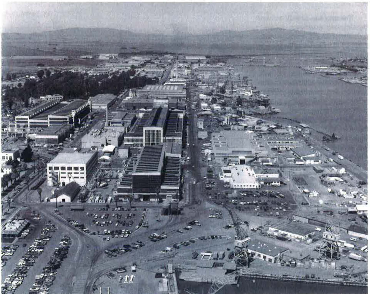
Aerial view of Mare Island's shipyard industrial complex looking north.
