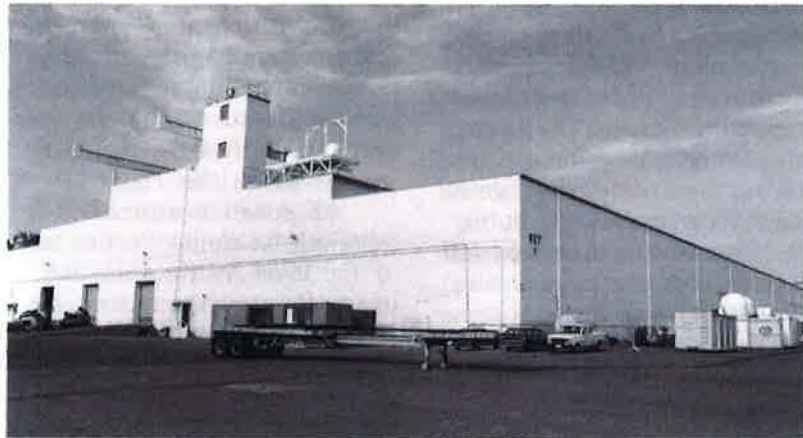
Warehouse Building 627, located on the north end of Mare Island, contains 220,000 square feet and can be easily converted for civilian use.
