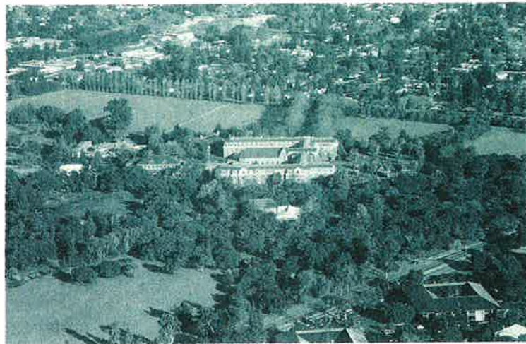
Some of the most prestigious areas of the country are on the other side of the Dumbarton Bridge in the Menlo Park and Palo Alto communities near Stanford University.
