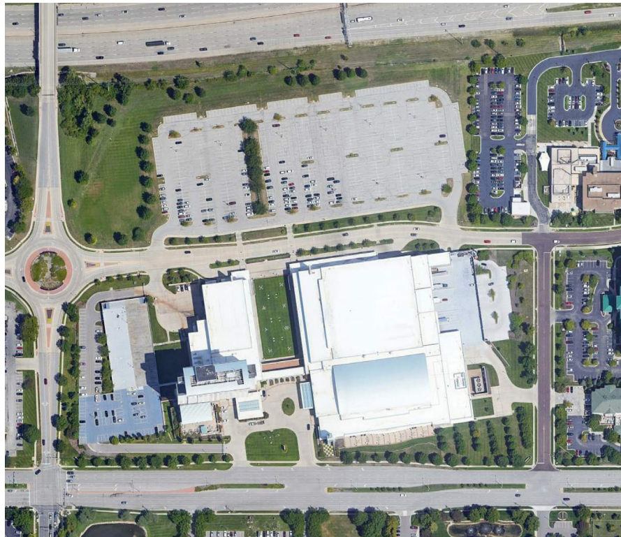
Aerial photo of the 10-acre study site, the Overland Park Sheraton Hotel.
