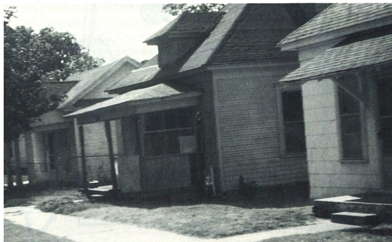
Many of the houses in Metro Park need repair.
