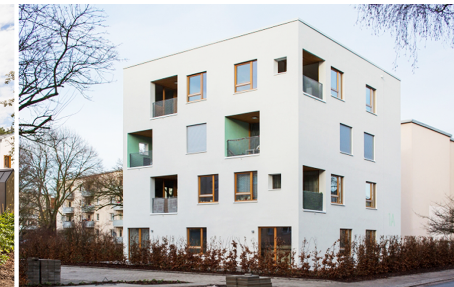
Prefabricated modular timber apartment bldg.
