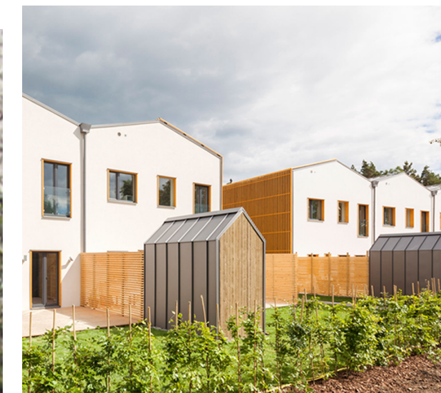
Zero energy row houses
