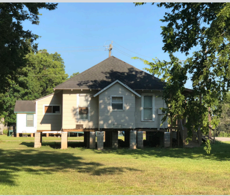
Some homes have been raised temporarily, awaiting final repairs or foundation work until a levee is constructed south of the neighborhood along the Colorado River. Source: ULI Houston.
