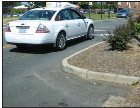
(Figures 12a & 12b) Bulb-outs can create a perceived narrowing of the road, which can help reduce vehicular speed.
