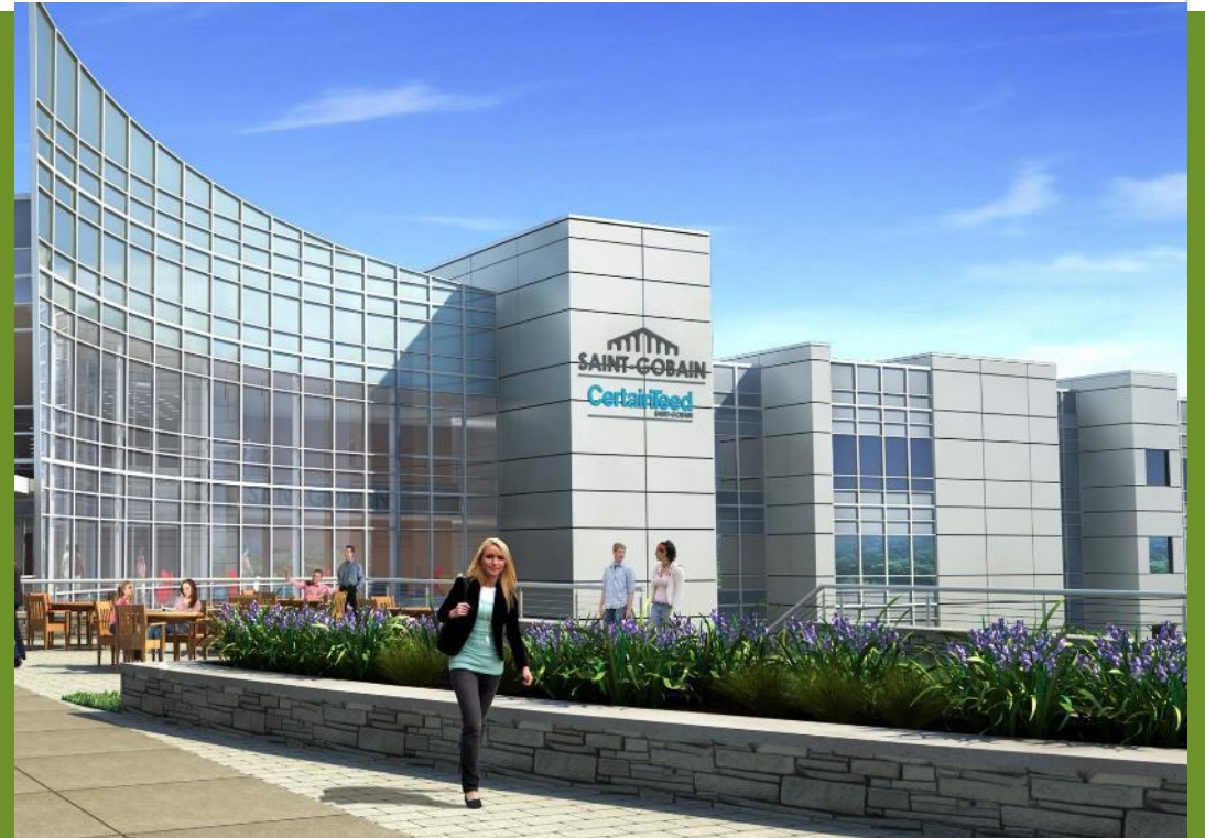
St Gobain, new LEED-Certified office with a focus on health
