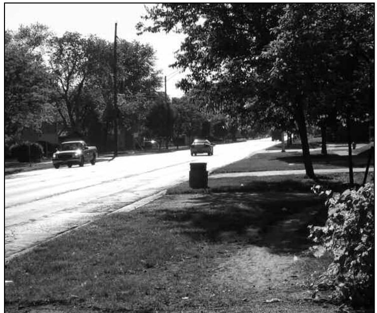
Figures 11 Sidewalks should be added to improve the environment for pedestrians.
