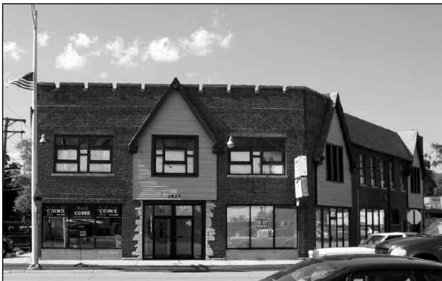
Figure 7 The Kreis building presents a wonderful opportunity for reuse in the village center.
