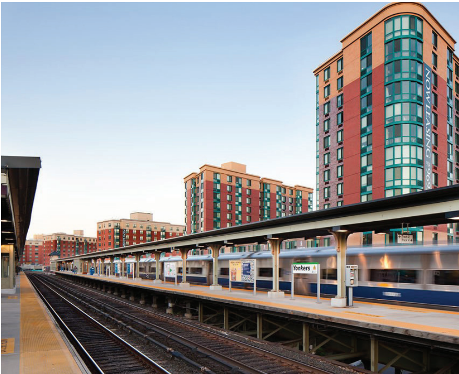
The Metropolitan Transportation Authority invested $43 million in renovating the 1911 train station building and platforms, as well as the reconstruction of the viaduct that carries the elevated tracks, construction of a mile-long retaining wall, and replacement of bridges.
