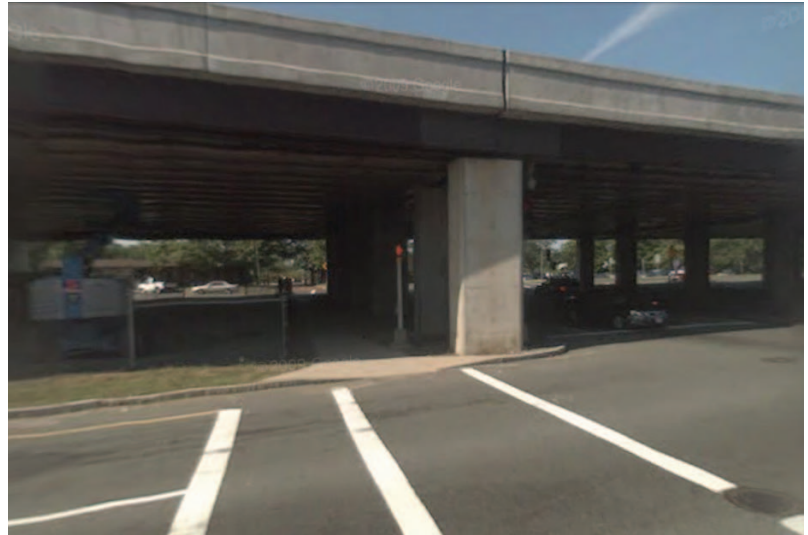
The pedestrian walk through the State Street underpass beneath I-91.
