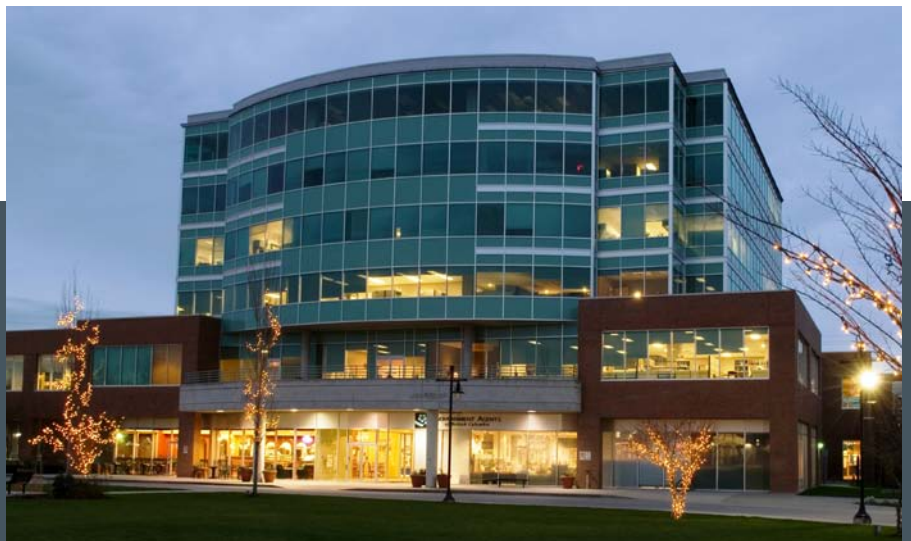
District of Maple Ridge Municipal Office
