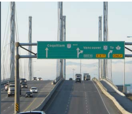
Pitt River Bridge
