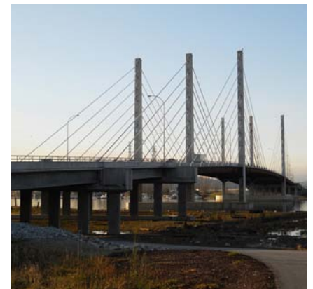
Pitt River Bridge
