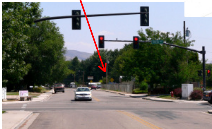
School crosswalk, looking from end of pathway
