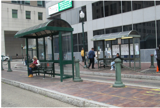
The Market Square area, where the Transfer Center is currently located, could be a handsome gateway for downtown Harrisburg.
