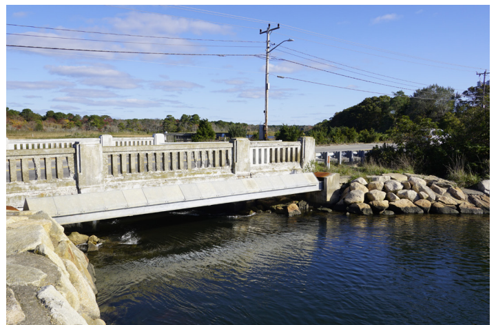
Parker's River Bridge
