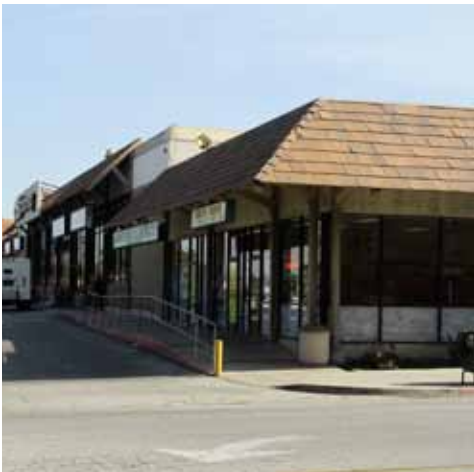
Implementing a low cost commercial rehabilitation loan program can promote effective use and reuse of smaller commercial buildings.
