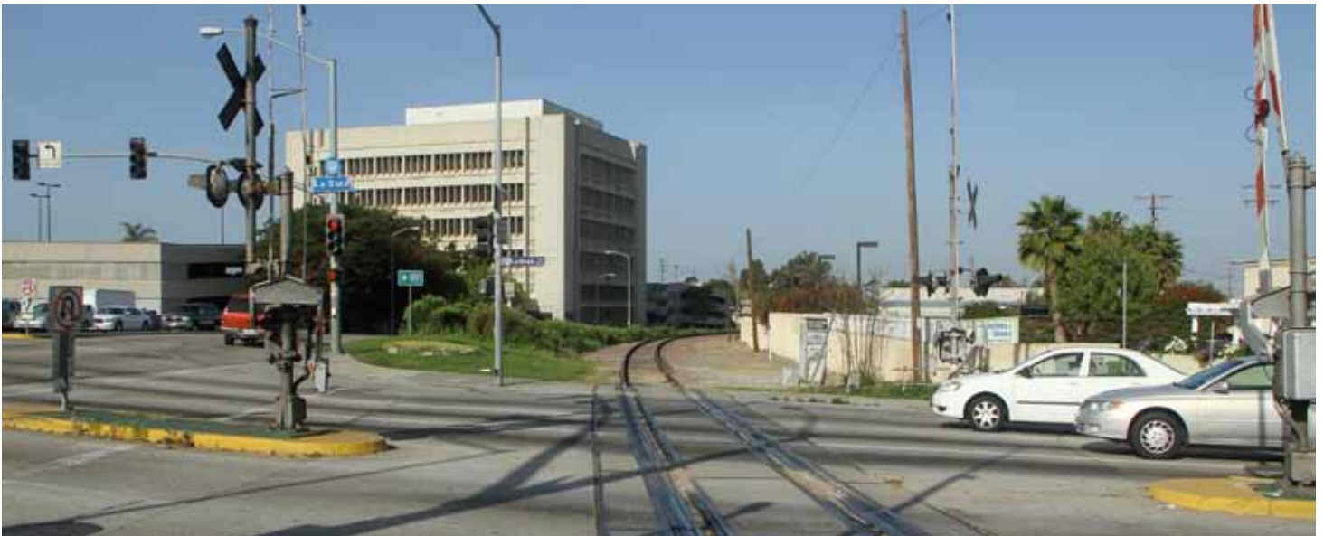
The new Crenshaw/LAX LRT will connect the Expo Line LRT from the Expo/Crenshaw station to the Green Line LRT at the Aviation/LAX station.
