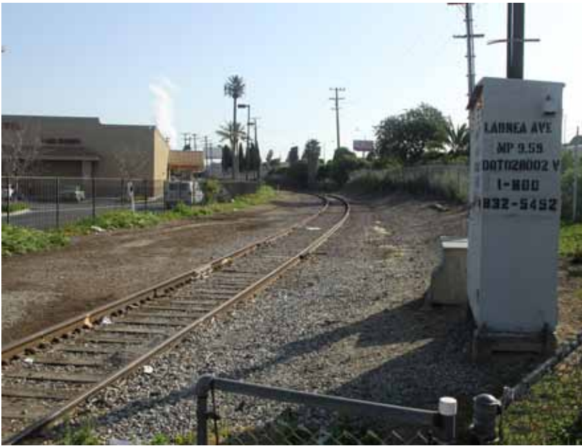
The proposed station would be located in the Burlington Northern Santa Fe (BNSF) railroad right of way.
